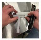
Cut off a small section of insulation for the short side of the drain tube as shown above.
