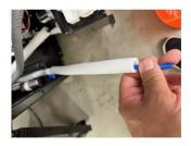
Locate the inlet water line to the filter bank and remove the insulation after the ball valve by simply slipping it off.
